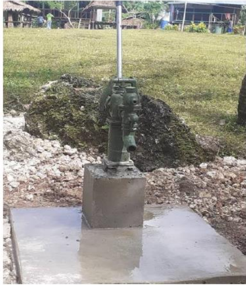
(a) Kaduwaga well water pump Completed on 12/4/21.
