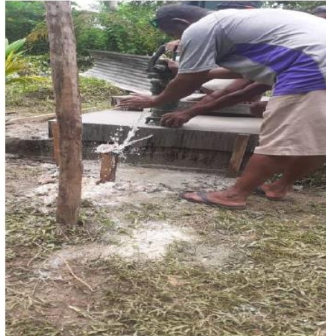
(e) Sinaketa pump testing
